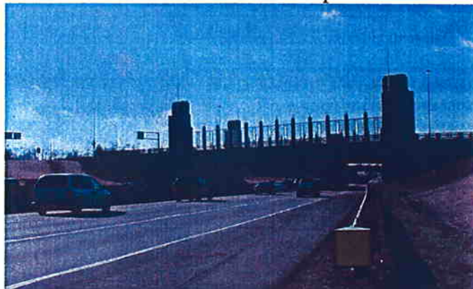
Recently completed Paddock Road bridge
