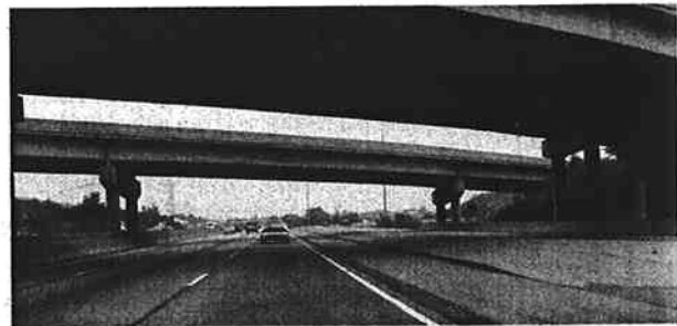
I-75 NB under SR126, showing proximity of bridge piers to I-75 existing edge of pavement.
