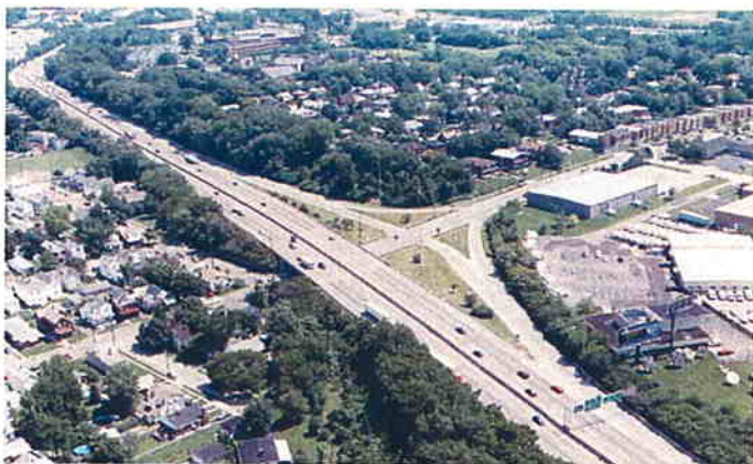
Towne Street Interchange (photo by Larry Stulz)
