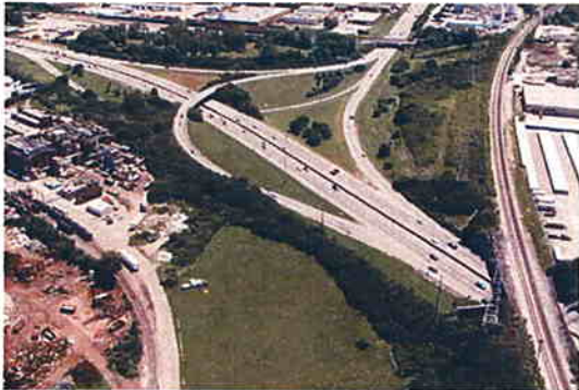
Norwood Lateral (photo by Larry Stulz)
